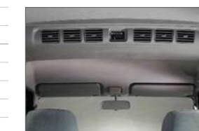
Dual Air Conditioning System
